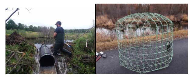
The upstream end of the leveler can be placed in a sunken cage made from livestock panel fencing. To extend the life of the cage, use epoxy coated wire mesh as shown in the right image. If holes are drilled in the water leveler it does not to be level. Tip: The farther the cage is from the dam the harder it is for beaver to determine the origin of the leak. With a plastic culvert use a minimum of one 20-footer. Photos by Ben Nugent, USDA-Wildlife Services
