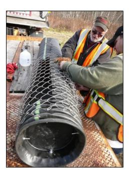
Culvert being modified to use either as a water leveler or culvert extension. Intake end is blocked with a heavy rubber livestock dish. They are available in many sizes.
