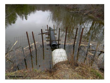
Arc-shape exclosure with channel post and concrete reinforcement wire. The leveler is made from a piece of salvage plastic culvert, with the end blocked and a slot on the underside to receive water. **NOTE**: Leave a gap on one side, between the first post and the shore if turtle passage is a concern.
