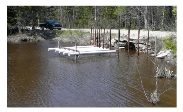
**3. Small-diameter plastic culverts**: Use like the perforated drainage pipes. Block the upstream end. Cut a long, narrow slot in the upstream end, wrap with light-duty fencing and place the slot towards the water. The intake capacity of the slot should exceed the opening of this culvert by 25%. This method affords high flow capacity and less support structure than needed with multiple perforated drainage pipes. These move water from upstream and through the inside of the exclosure.
