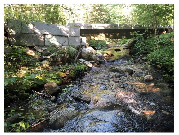
This crossing is constructed with commercially available modular concrete blocks. It is greater than full bank width and retains the natural substrate. Photo by Chuck Hulsey, MDIFW
