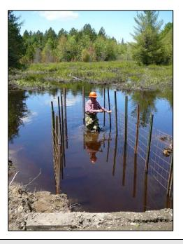
Beaver are hard-wired to build *perpendicular* to the waterflow, so having a large percentage of the exclosure perimeter aligned parallel to the water course is meant to "deceive" them. This design was developed by wildlife biologist Skip Lyle.
