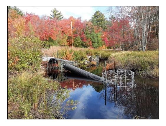
Exclosures are constructed with livestock panel fencing. Both were built on dry ground nearby. The white-tipped T-Posts were put in place with a light, hand-held fencepost pounder. Photo by Chuck Hulsey, MDIFW
